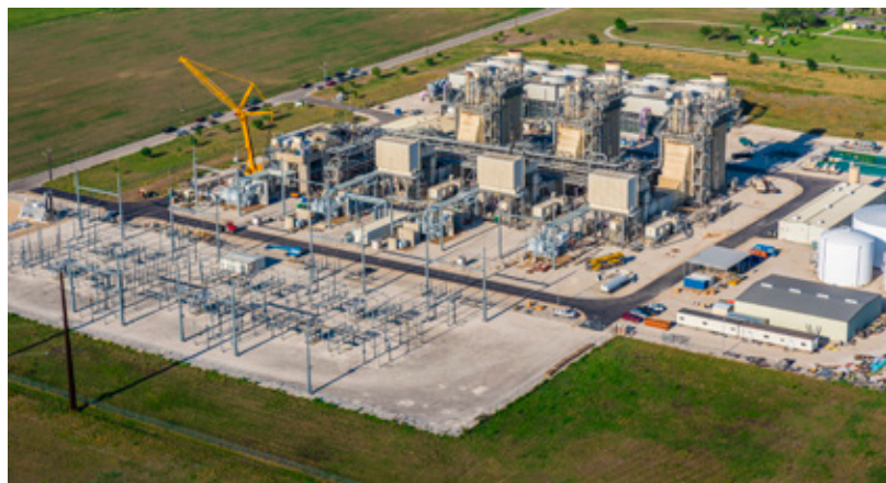
Natural Gas-fired Turbine Electrical Power Plant
